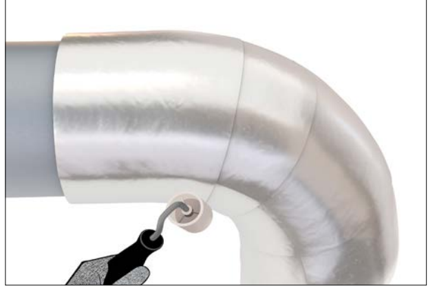
Figure 69: Securing overlaps with roller
