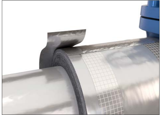
Figure 43: Application of vapour barrier tape at termination
