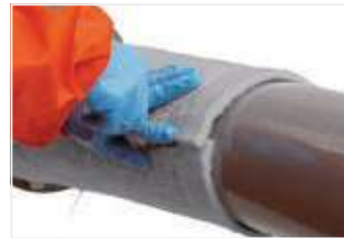
Figure 12: Longitudinal overlapped seam.
