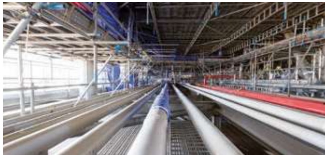
Figure 9: If adverse weather is likely, provide cover for work areas. Prevent insulation becoming wet.
