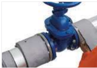
Figure 54: Wrap strips of ArmaGel HT around the pipe until the insulation exceeds the outside diameter of the flange.
