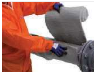
Figure 24: Ensure starting point is in line with axis of pipe. Tape or adhesive may be required to help hold the axial position.
