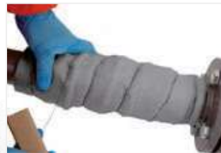
Figure 29: Spiral wrap with wire to hold ArmaGel HT in place.
