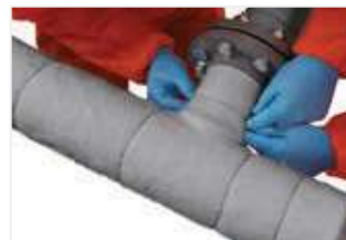
Figure 49: Wire into place.
