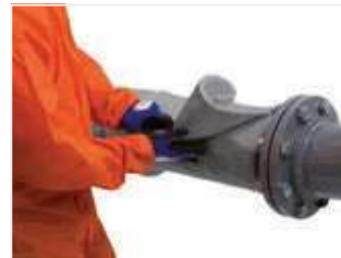
Figure 25: Continue to wrap around the pipe to achieve the required quantity of layers. End the wrap with the longitudinal edge in line with, or overlapped with, the inner layer starting point.
