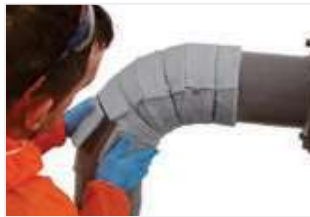
Figure 36: Wire each gore in place allowing movement for final adjustment.
