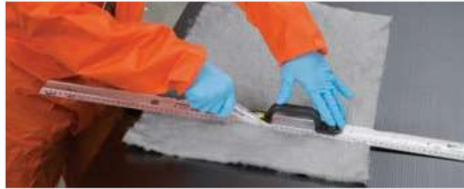
Figure 4: Prefabrication cutting in the workshop.
