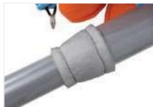
Figure 44: Fit around reducer and wire in place.
