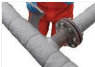
Figure 48: Install branch piece.
