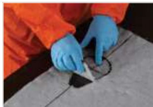
Figure 50: Create cut out for oblique angled branch.
