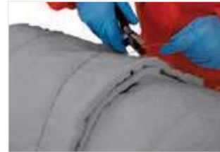
Figure 33: Wire in place.
