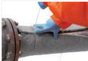
Figure 13: Start to bring together longitudinal seam and secure with wire.
