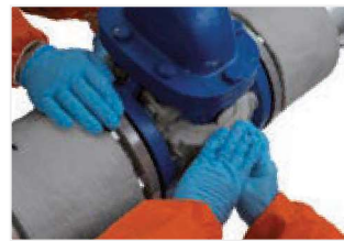
Figure 55: Pack ArmaGel HT around body of valve to prevent voids.
