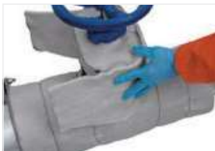
Figure 58: Wrap valve stem.
