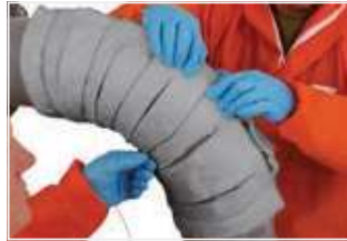
Figure 40: Push all gores together to ensure there are no gaps at joints or voids.
