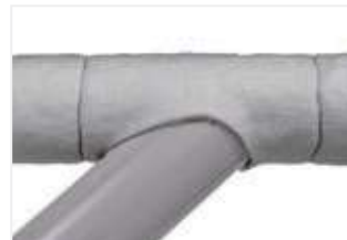
Figure 51: Wrap around pipe and wire in place.
