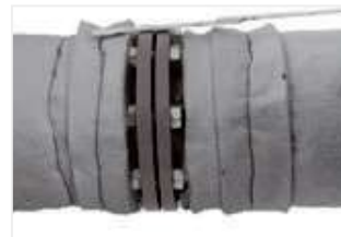
Figure 31: Wrap 50 mm (2 in.) wide strips of ArmaGel HT to build up insulation to clear flange (or adjust width to be equal to total insulation thickness if > 50 mm).
