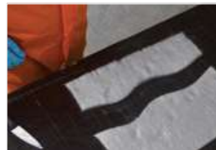
Figure 47: Cut shaped piece for branch.
