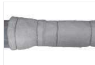
Figure 45: Butt pipe insulation tightly up to reducer.
