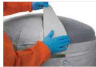
Figure 61: Apply closely-butted segments and fix using insulation stick pins and bands.
