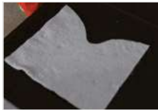
Figure 52: Cut material to fit the oblique angled branch.
