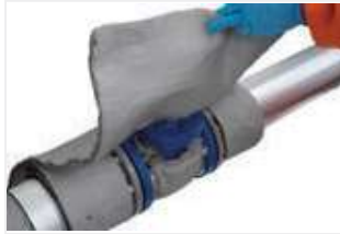
Figure 56: Wrap ArmaGel HT around flanges.
