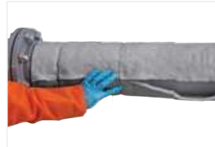
Figure 14: Continue to make seam, closing gaps.
