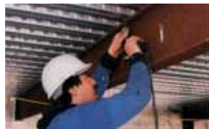
Fixing stud welded pins
