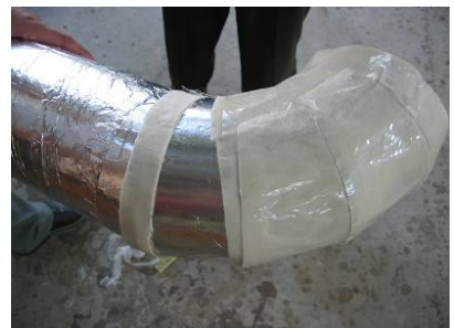
An elbow showing two lobster back pieces attached
