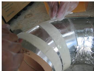
The strips of FibaRoll that go beneath the lobster back pieces. Note that the top film has been stripped
