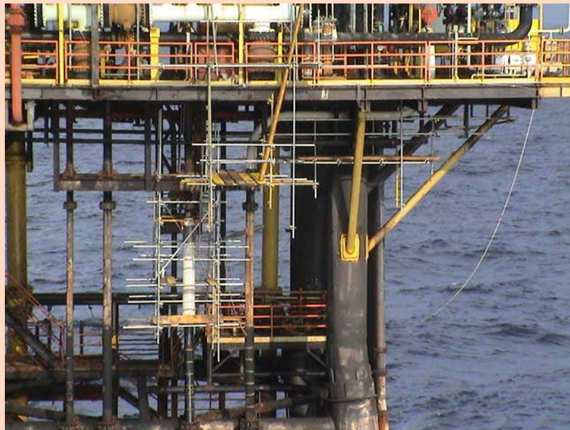
FibaRoll protecting corroded risers
