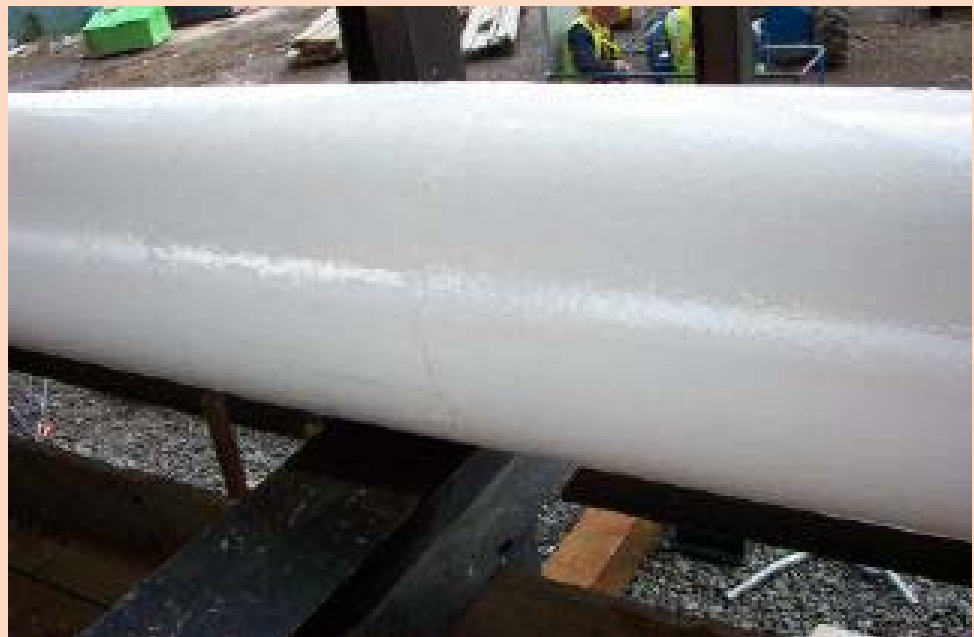
FibaRoll protecting main line coating from damage at pipe supports
