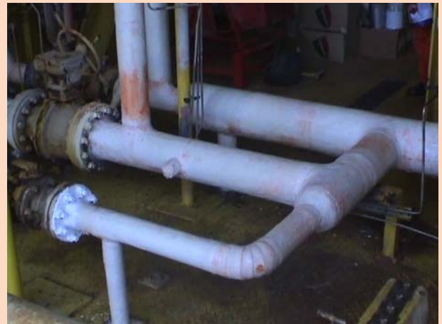
FibaRoll/FibaGel applied
