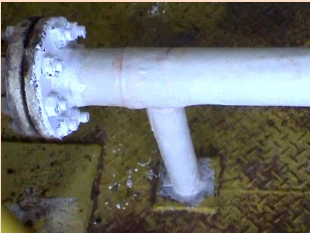
FibaRoll/FibaGel applied
