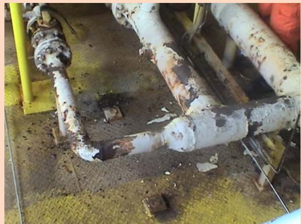
Corroded pipes
