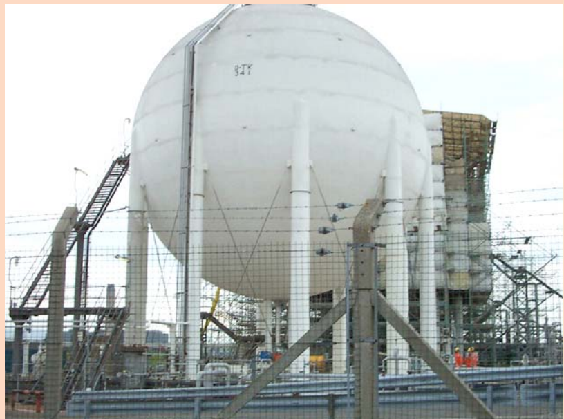
FibaRoll cladding on LPG spherical tank - Scotland
