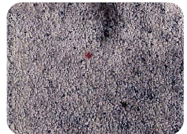
Another wet felted mineral fibre tile showing micro-organism growth
