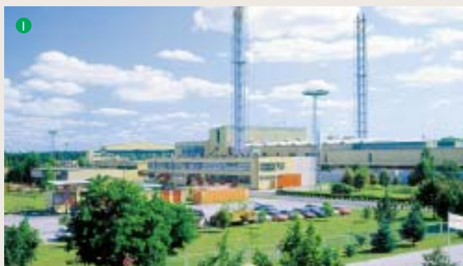
1 Energy efficiency improvements of 50% per production unit have been achieved when newly acquired factories are modernised with Rockwool know-how. Rockwool Polska has twice been awarded Leader of Polish Ecology.
